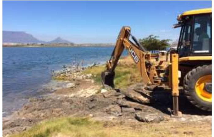
**Figure 44. Digger-loader removing the broken slipway near the public ablution block.**
