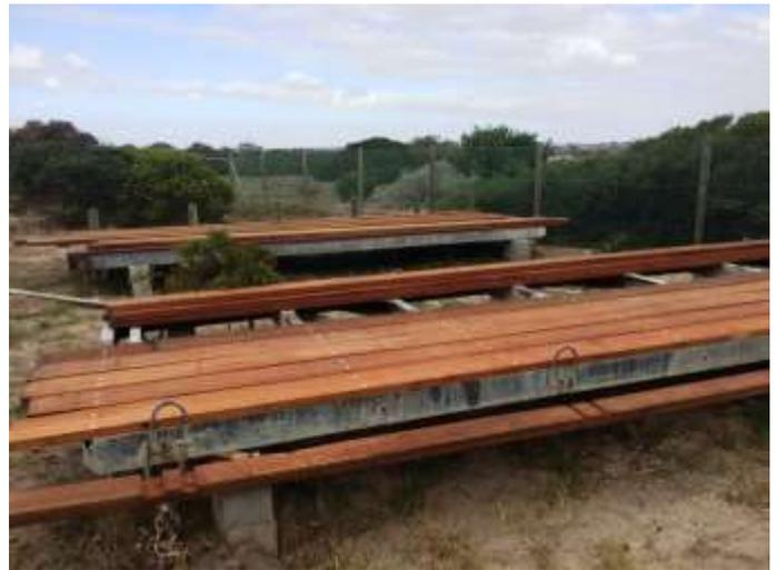
Figure 35. New timber on the old jetty.
